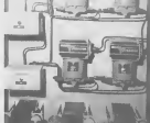
MOORE SQUARE root extractor is used in conjunction with analyzer control of units.
